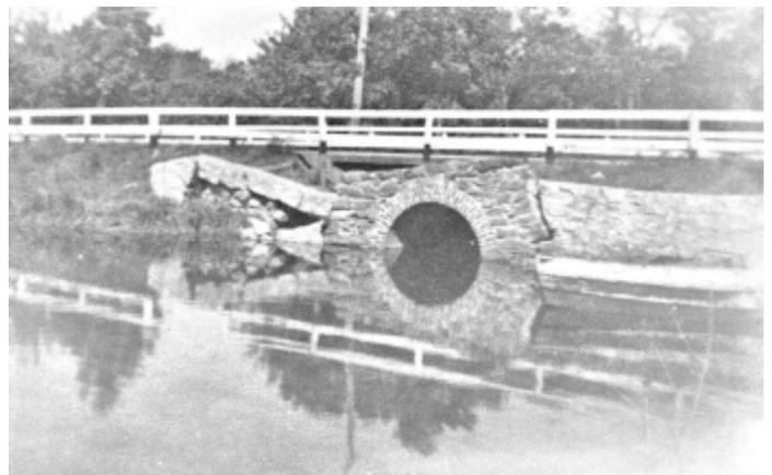
The stone arch bridge, reconstructed in 1931 when the roadway was concreted, only lasted for seven years. It was badly damaged in the 1938 hurricane and had to be replaced. Note the white fence railings. This view is probably of the south side of the bridge. The replacement bridge, finished in 1939, was of a more "modern" box culvert design, with stone railings. [This 1939 bridge was reconstructed in 2013.](#)
